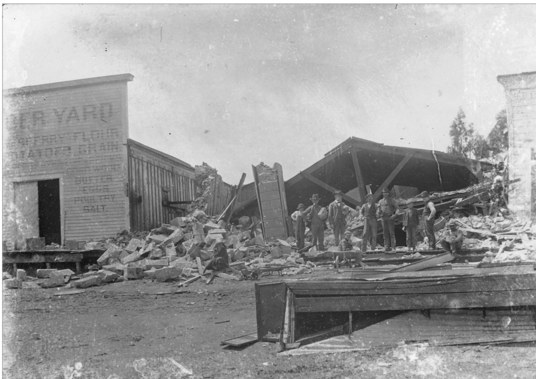
Holland's General Store, built of stone in the late 1850s by Warren Dutton, was demolished by the 1906 earthquake, along with four other Tomales masonry buildings. In one of these—a stone house on today's Sartori Ranch—two children were killed, and one died several years later of her injuries. In some cases, the concept of “recovery” is only relative. (photo by Ella Jorgensen)
