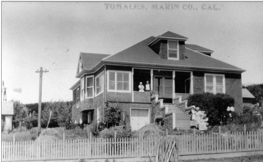
The shingled Cornett-Diekmann House on Railroad Avenue at Second Street in Tomales — the home of two well-known families of local merchants. (photo by Ella Jorgensen)
