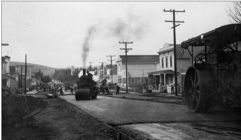
This first-ever paving of a Tomales road must have been a memorable mark of Progress. Ella Jorgensen captured this view and several others of Maine Street being paved in the mid-1920s. View south on Highway One; Dickinson Store (now Diekmann’s) and Post Office at center.
